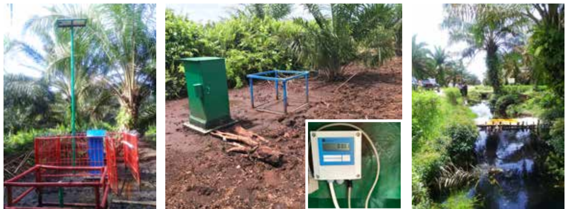
Ground Water Level (TMAT) Monitoring using data logger
